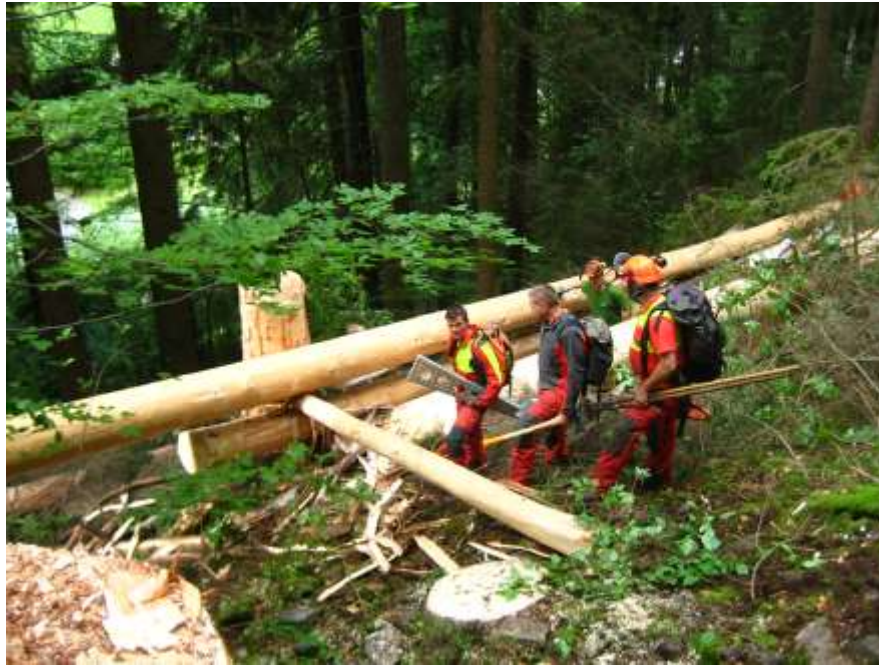
Figure 16: Example of a structure made by stacking logs.
