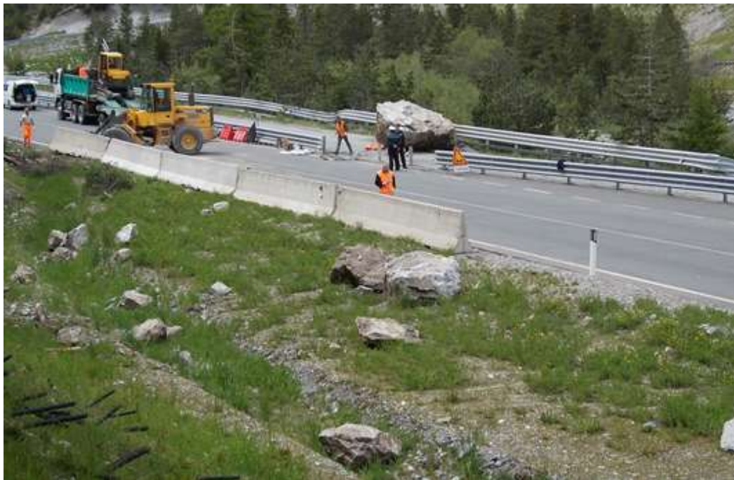
Figure 68: Removal operations for the boulder fallen on SS24 road during June 2011.
